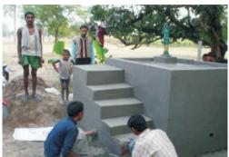
during floods ,10 raised hand pumps have been installed in the area with 6ft height and boring level up to 80 fts long with platform and staircase on it. Hamlet development committees are regularly monitoring and maintaining the hand pumps.
